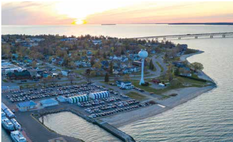
Enbridge's Line 5 runs under Michigan's Straits of Mackinac en route to Sarnia, Ontario from Superior, Wisconsin. Line 5 feeds regional refineries in Ontario, Michigan, Ohio, Pennsylvania and Quebec. The pipeline serves Sarnia's refining complex, providing gas and jet fuel to some of Canada's busiest airports, and supplies Quebec's refineries with about 60 percent of their feedstock. —Enbridge photo
