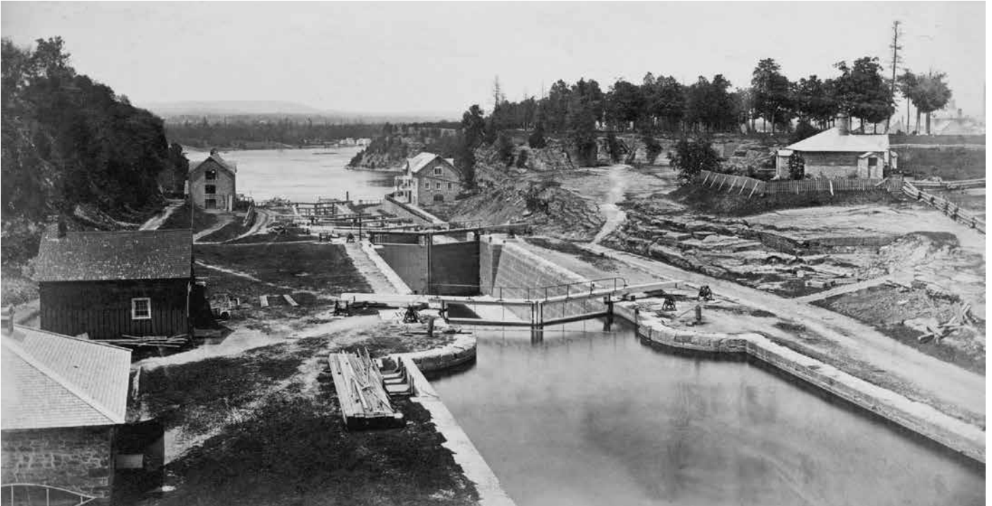
The Ottawa Locks of the Rideau Canal in 1869, showing part of the quarry on the east side where Mackay was able to extract superior seams of limestone. —William Notman, McCord Museum I-38066.
