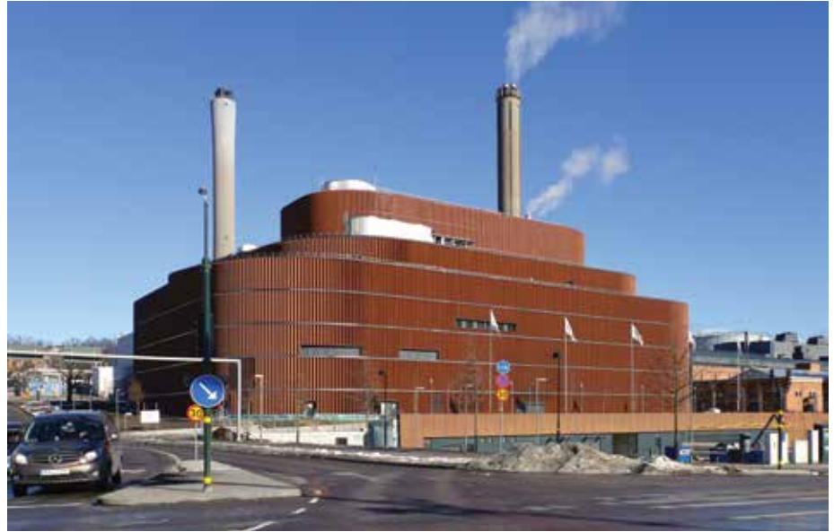
The wood chip-fuelled KVV8 combined heat and power plant in Stockholm —Holger Ellgaard
