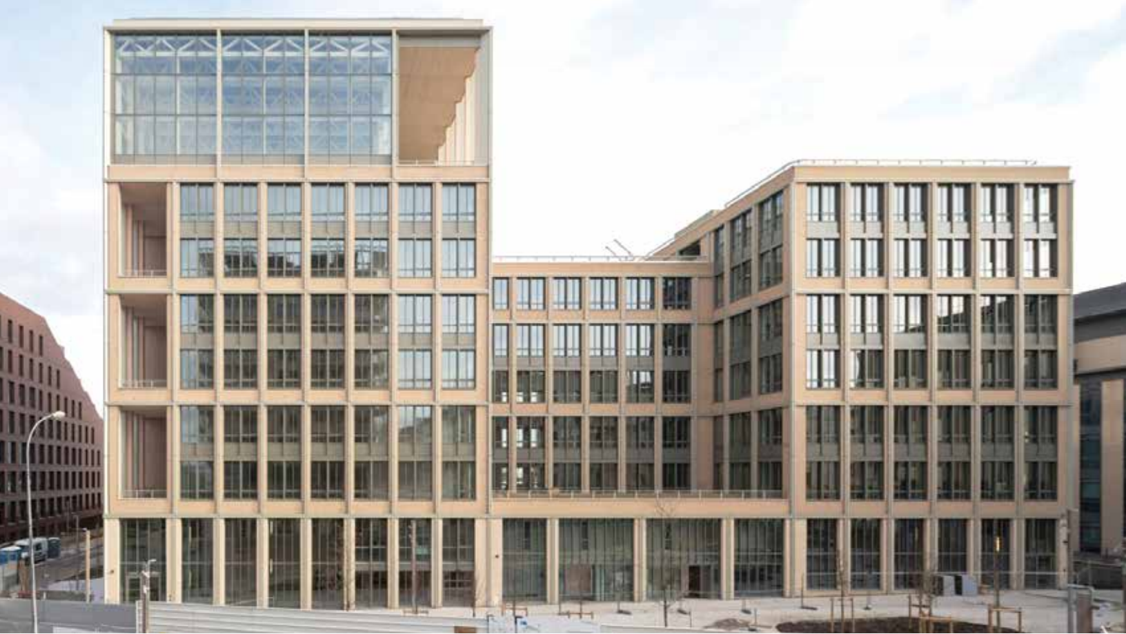
The mass timber office building in the Paris Olympics Athlete's Village —Dezeen
