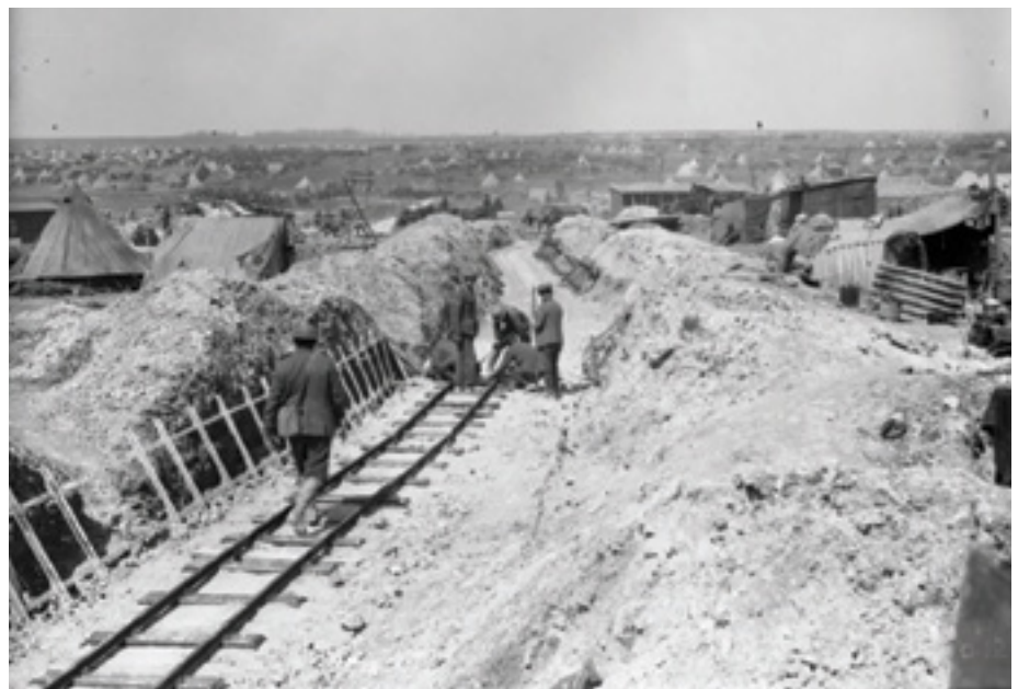
Canadian railway workers build a railroad through captured territory during the Battle of Vimy Ridge in April 1917. Photo: Canada. Dept. of National Defence / Library and Archives Canada
