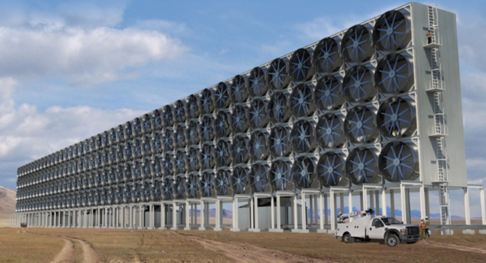
An artist's depiction of a Carbon Engineering 'air contactor slab' that would capture 100,000 tonnes of CO 2 per year and turn it back into fuels like gasoline or diesel in a process called air to fuels (A2F). Carbon Engineering photo
